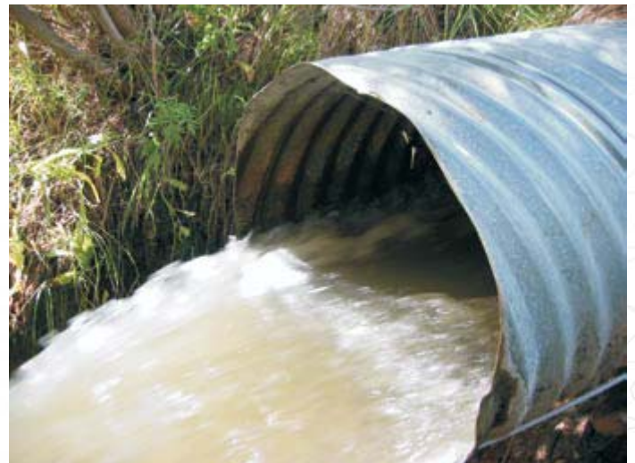
Lafarge Lagoon Discharge
